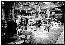
Desalters will treat up to 20 million gallons a day of water with high total dissolved solids and nitrate levels. The desalters will increase local water supplies by making previously contaminated water available for use, and will help lower groundwater levels, preventing water from rising and spilling into the Santa Ana River, where it would otherwise be lost to downstream communities.
